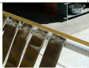
Use metal screws and washers to attach the fire hose to the metal poles. The space between fire hose pieces should be about 1 inch.
